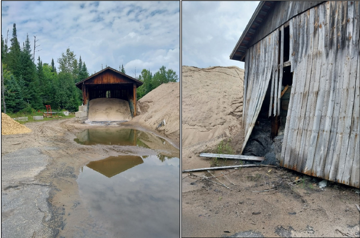
Figure 1. Salt Storage Facilities
